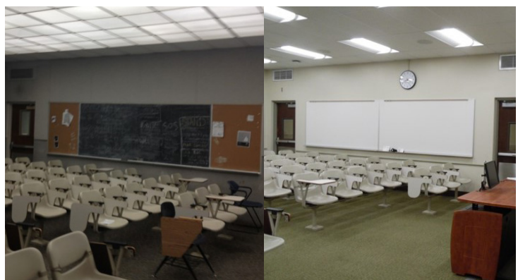
Olson Hall classroom before (left) and after (right) renovations.
